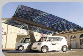
Photovoltaic shade structure for electric car
